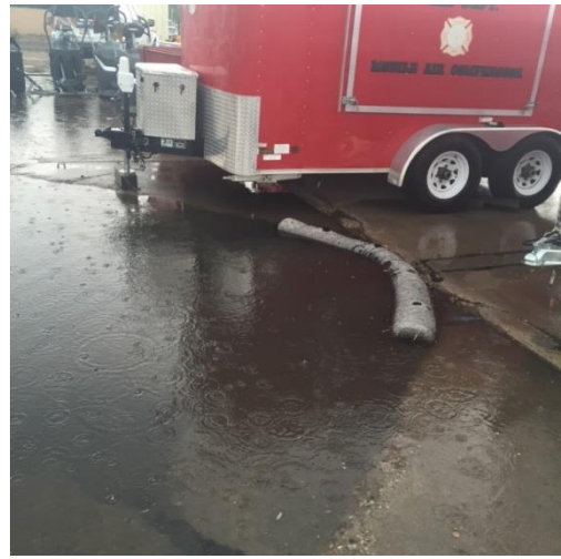
FM2 Ponding inside site
