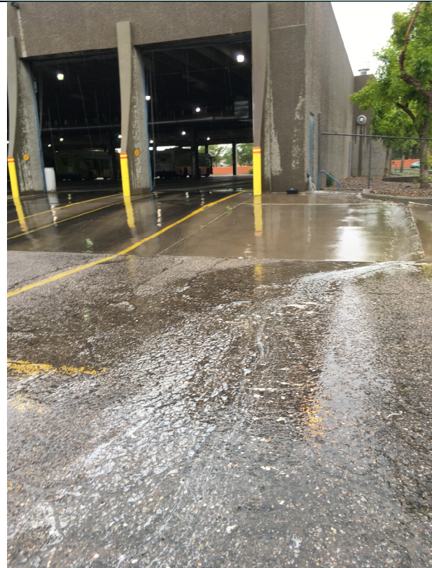
Photo 2: Some foam observed in runoff from roof drain.
