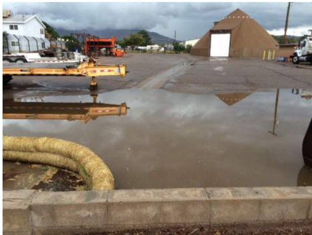
Ponded water observed near outfall.
