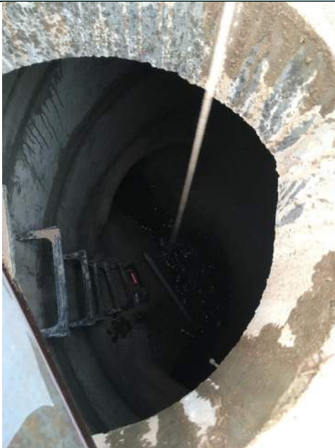
Outfall D2 – Bailer used to retrieve stormwater sample for visual observation.
