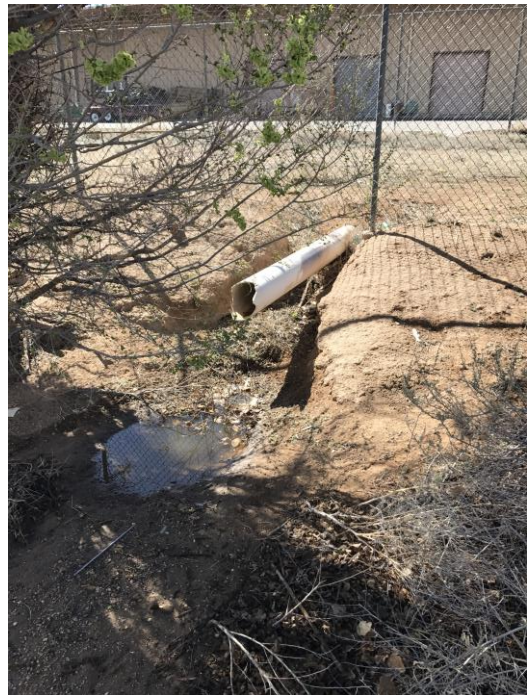
Took sample from pooled water at outfall MP1
