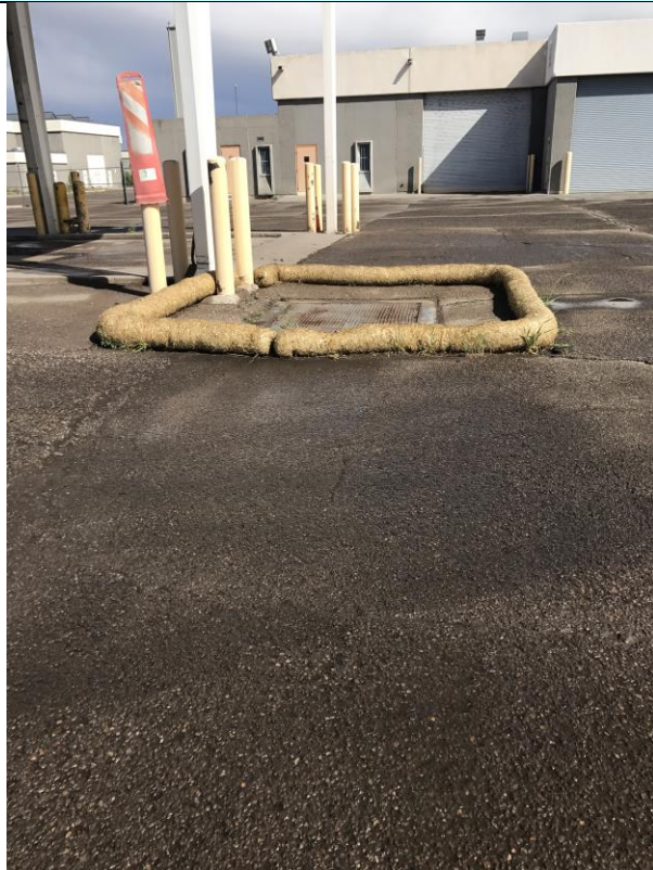
Photo 1: Water trail leading to outfall SS1B
