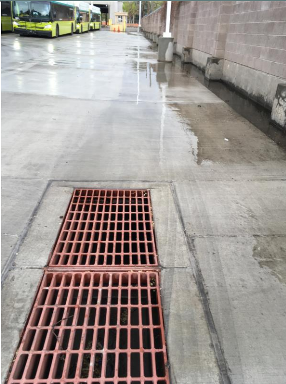
Photo 1: Inlet near bus fueling.
