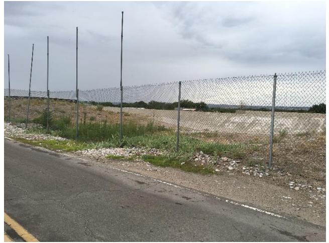
No discharge observed
