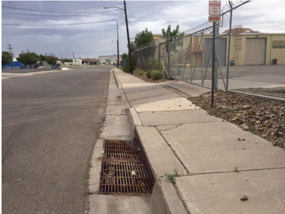
No discharge observed
