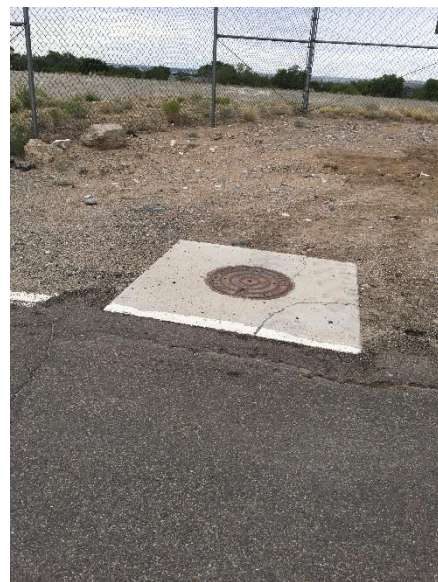
No Discharge Observed
