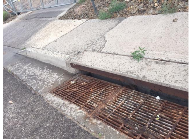
No discharge observed
