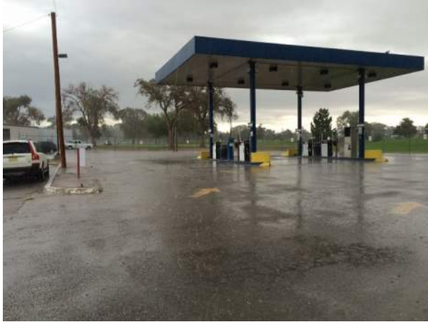
Runoff observed at Lomas Fuel Station
