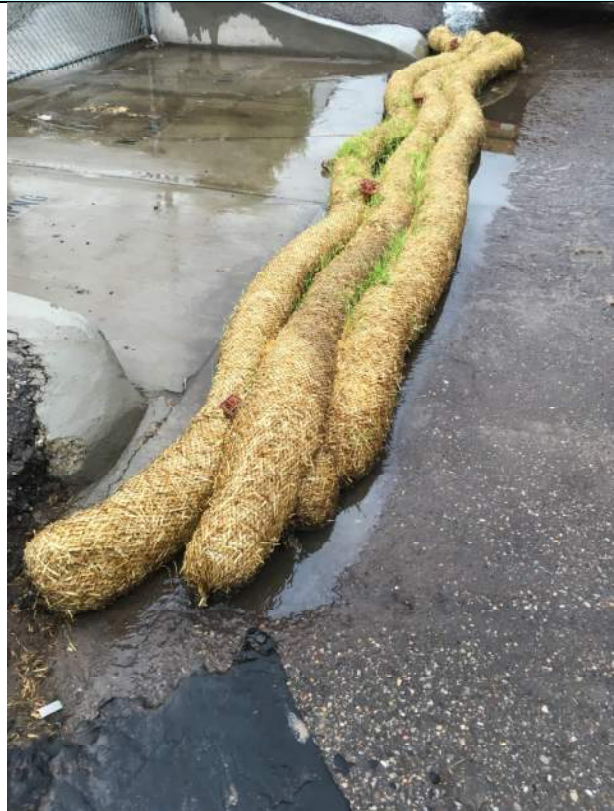
Wattles installed upstream of outfall.
