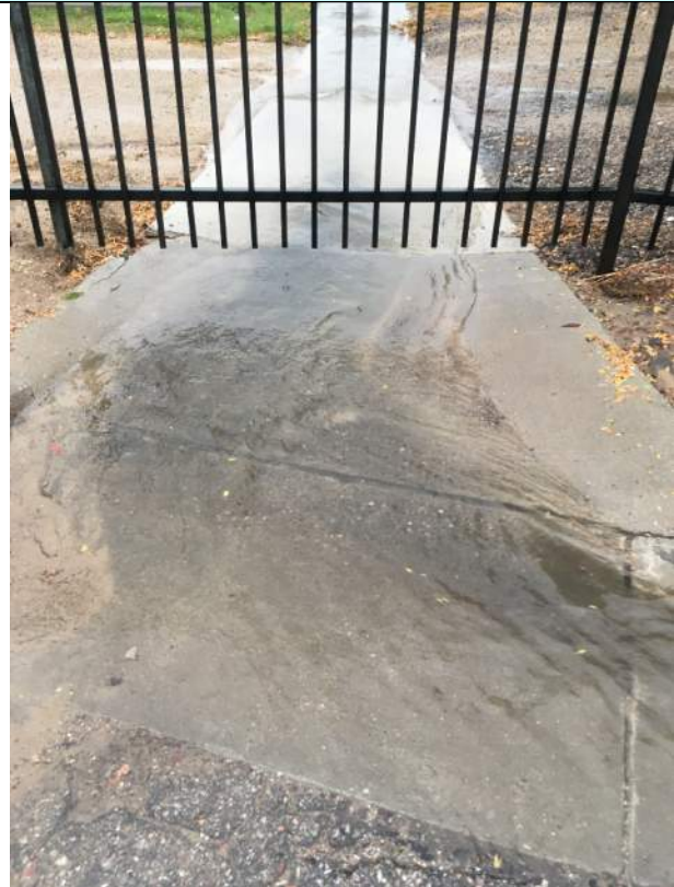
Runoff to Outfall LGC2
