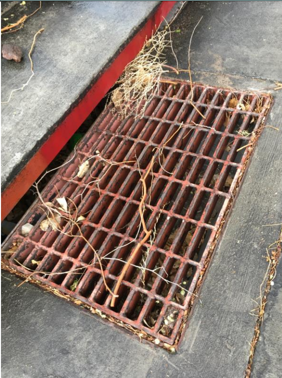
Photo 1: Leaf and other litter observed in PDS1 inlet.
