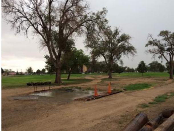
No runoff observed by golf maintenance wash pad.
