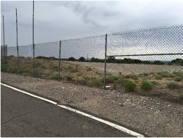
No discharge observed
