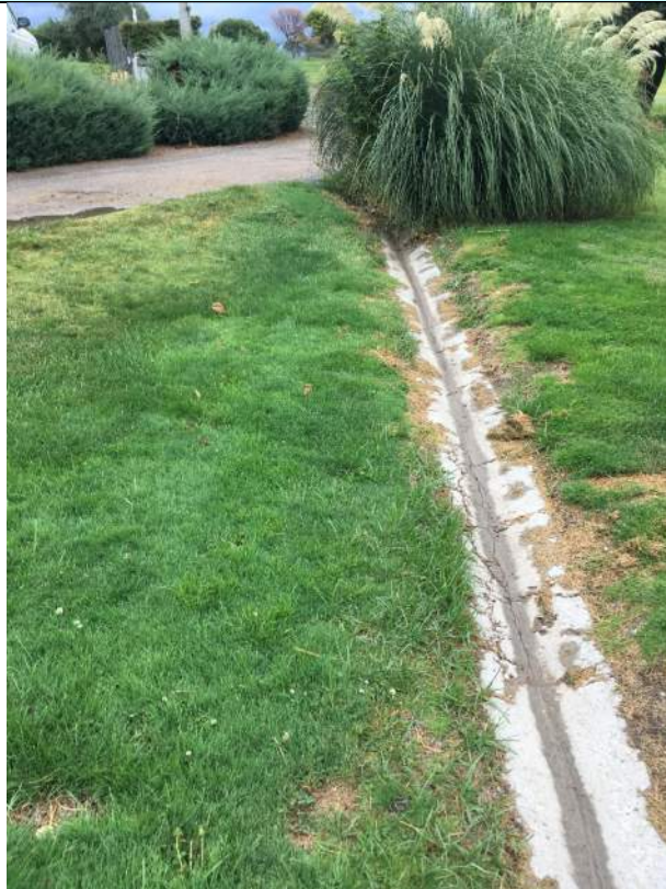
Concrete curb from maintenance area to outfall.
