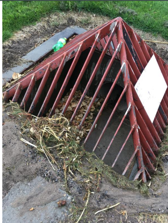
Photo 2: Leaves, sediment, and grass clippings in outfall PDS2.
