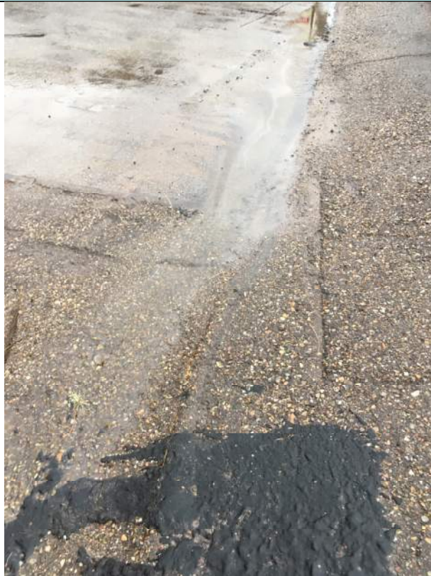
Sheen observed in runoff upstream of outfall.
