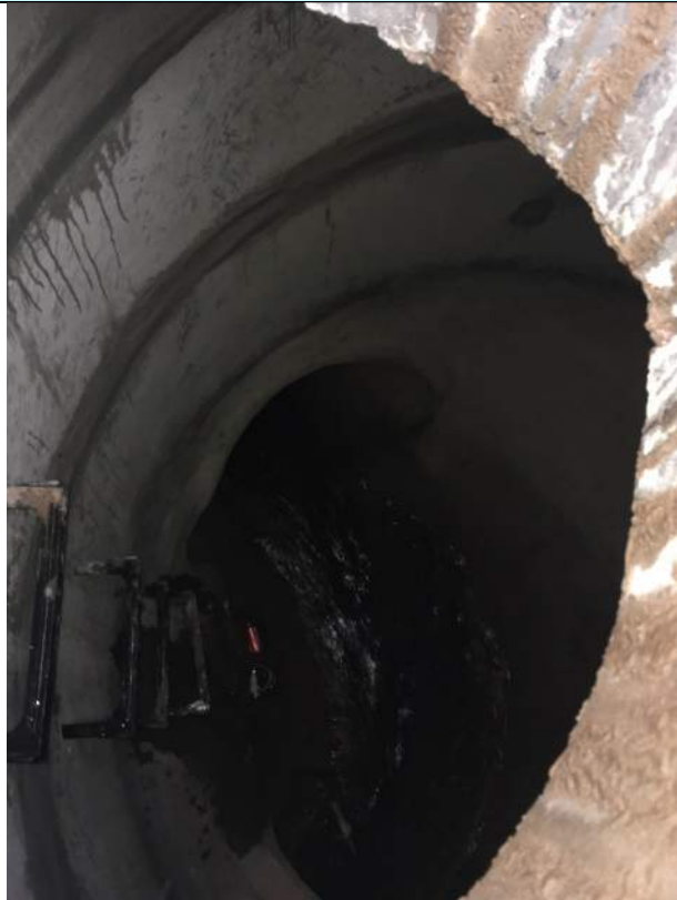
Flow observed in Outfall D1.
